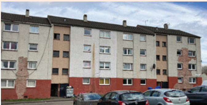
Flats before the work is carried out
