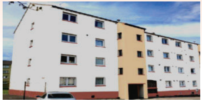
Flats after work is carried out
