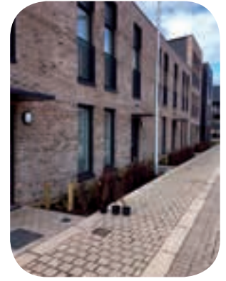
New homes at Capella Gardens, Greendykes
